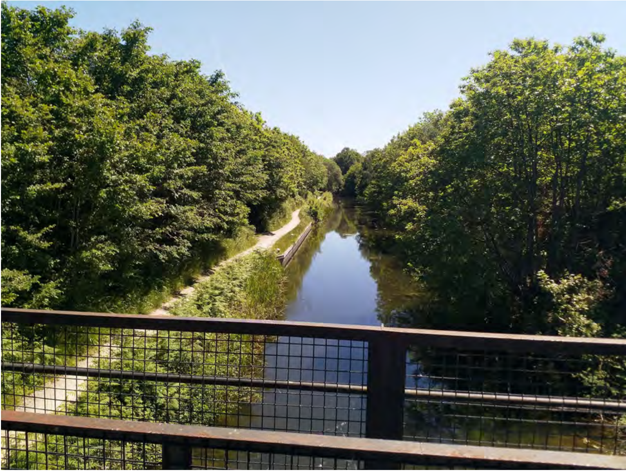
Image 7—View to the East into sub area from Eelmoor bridge
