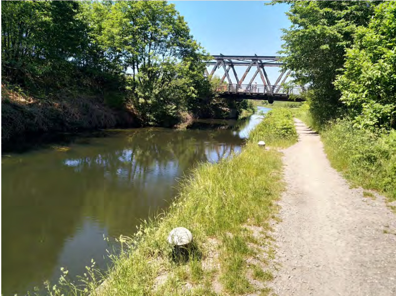
Image 8—View to the West looking towards Eelmoor Bridge
