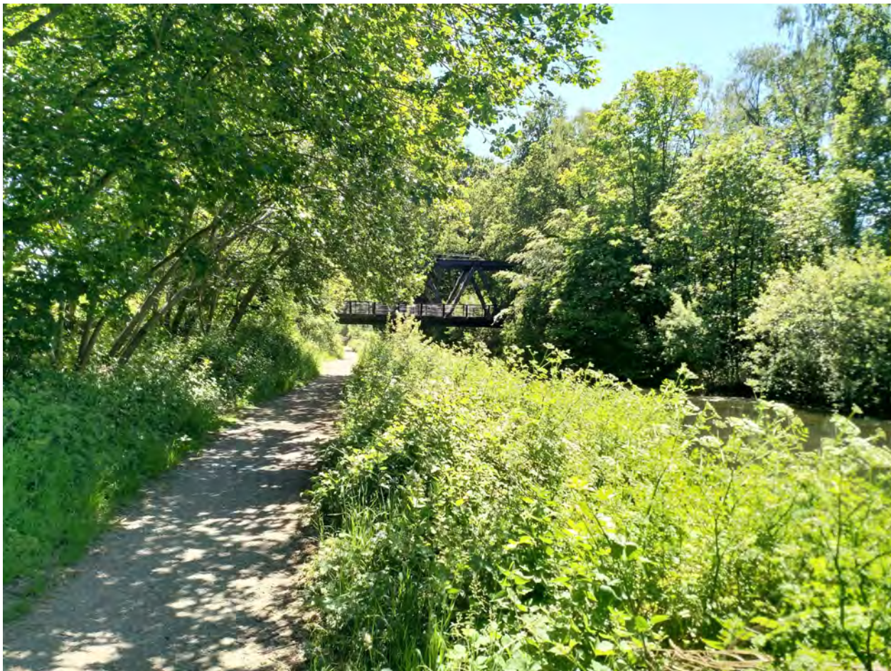
Image 11—View Eooking East towards Claycart Bridge
